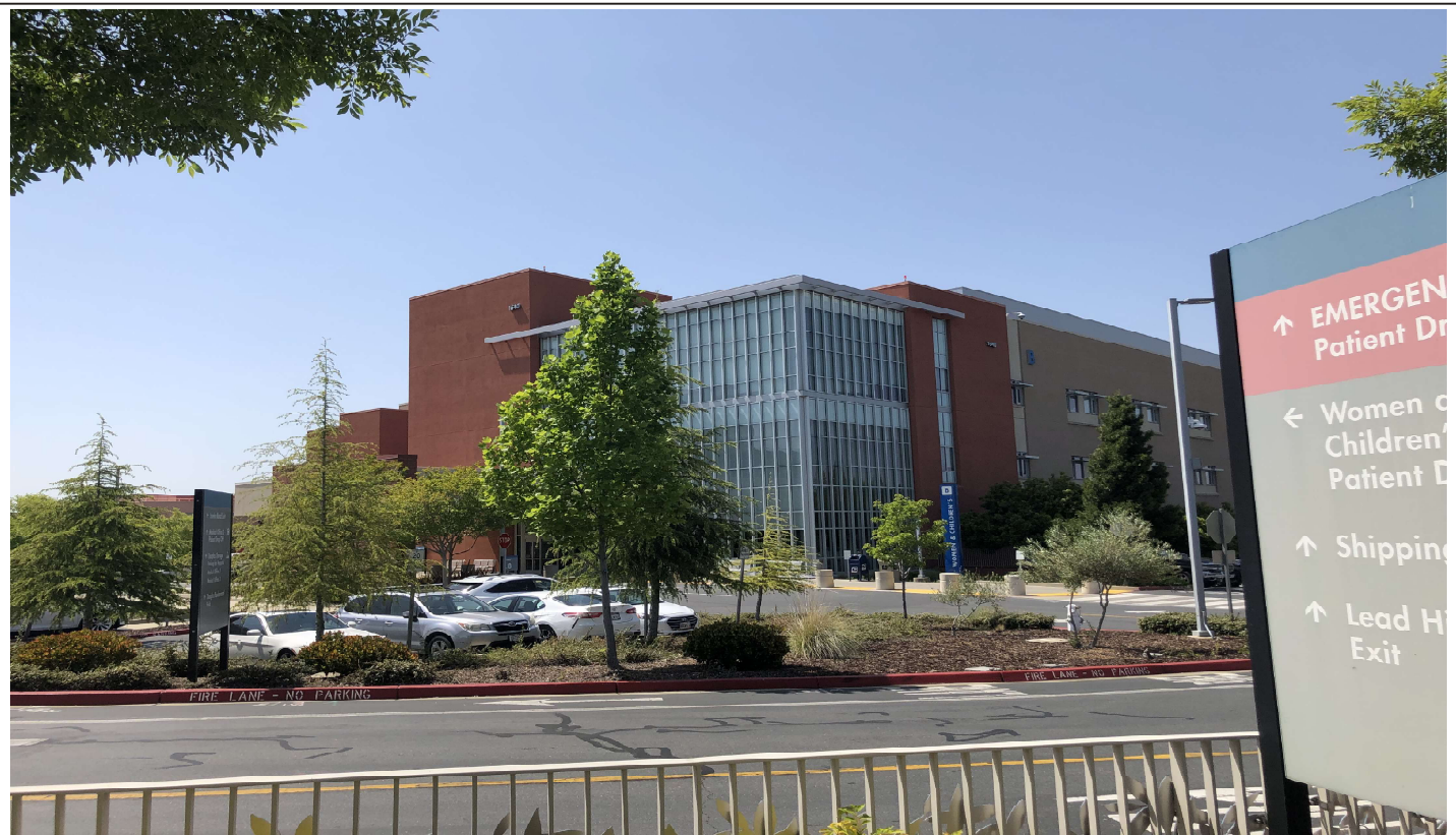
Viewpoint 9: From the Eureka Road entrance, looking northwest at the Woman's and Children's Center Building.
